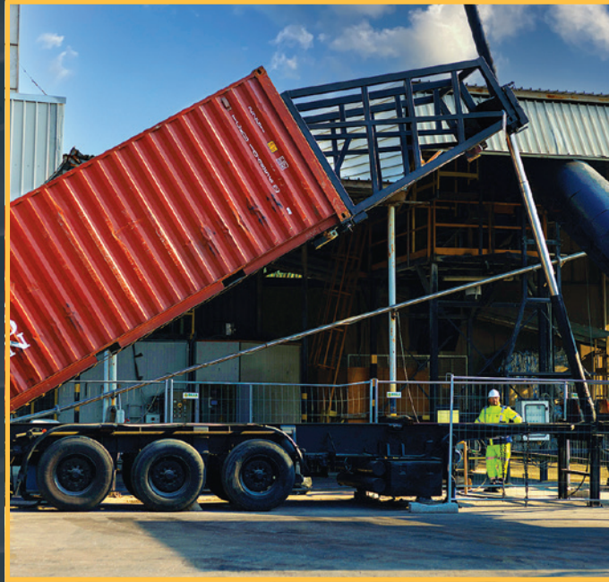
Bulk being unloaded into transfer silos to pack 25 kg bags or big bags
